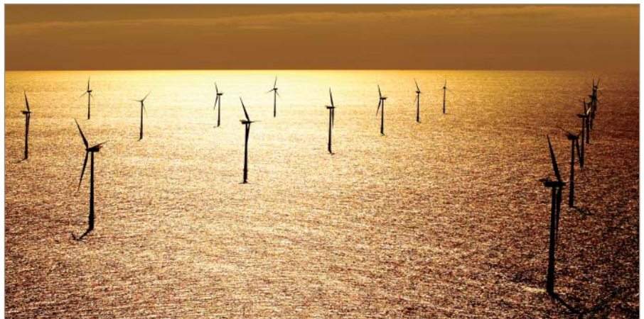
Fig. 1. Completed in December 2003, Nysted offshore wind farm in Denmark has 72 turbines with a total capacity of 166 MW, making it the world's largest (copyright: Elsam A/S)
