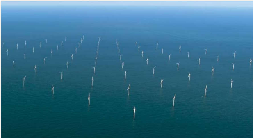
Fig. 4. Horns Rev wind farm has 80 turbines generating 160 MW (copyright: Elsam A/S)
